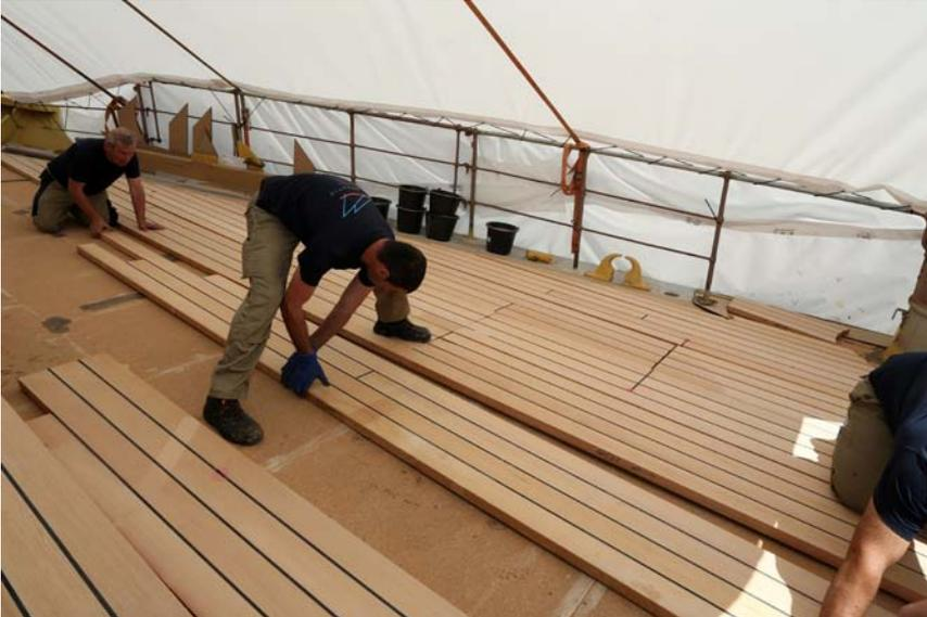
Precisely prefabricated deck plank elements are laid on the forecastle deck
